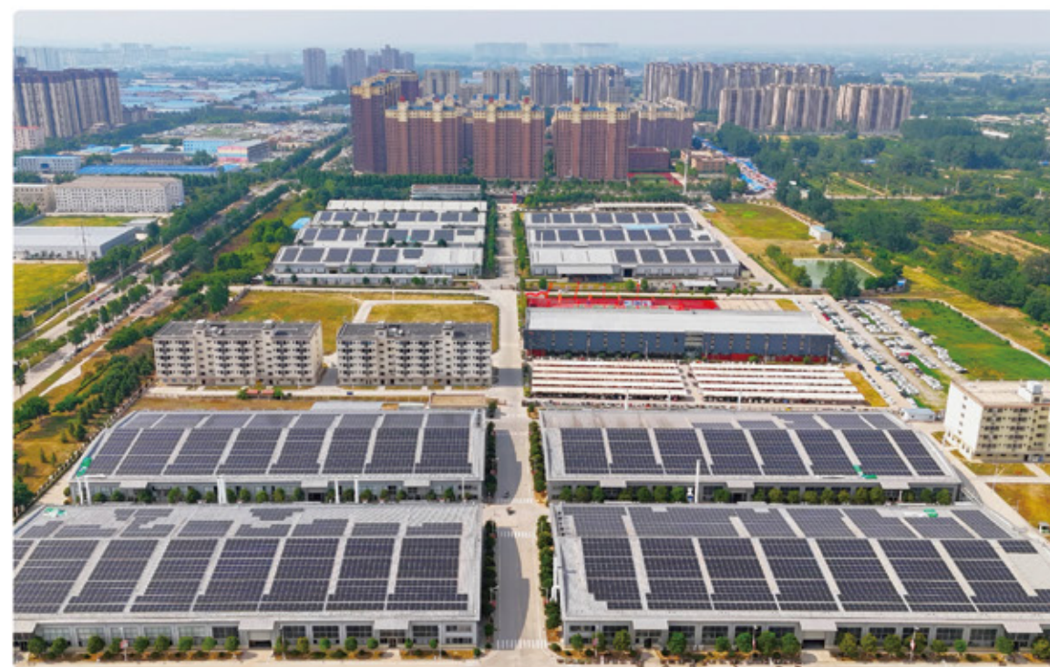
安踏6.4MW工商业光伏电站 Anta 6.4MW Commercial PV Power Plant
