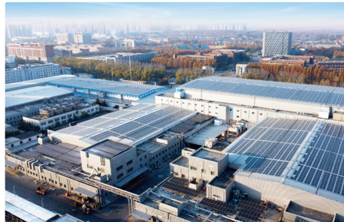
思念食品4.4MW工商业光伏电站 Syneer 4.4MW Commercial PV Power Plant
