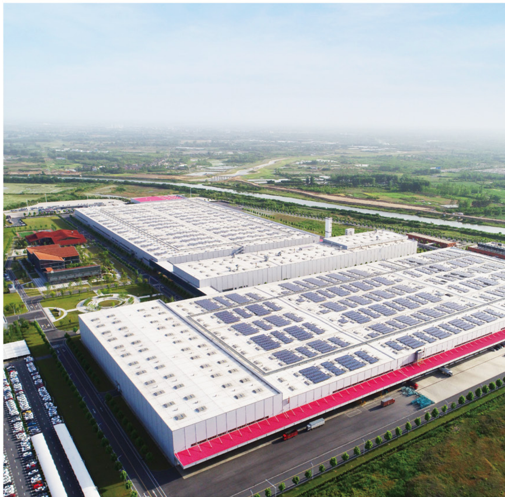
蔚来汽车先进制造基地5.028MW工商业光伏电站 NIO Advanced Manufacturing Base 5.028MW Commercial PV Power Plant
