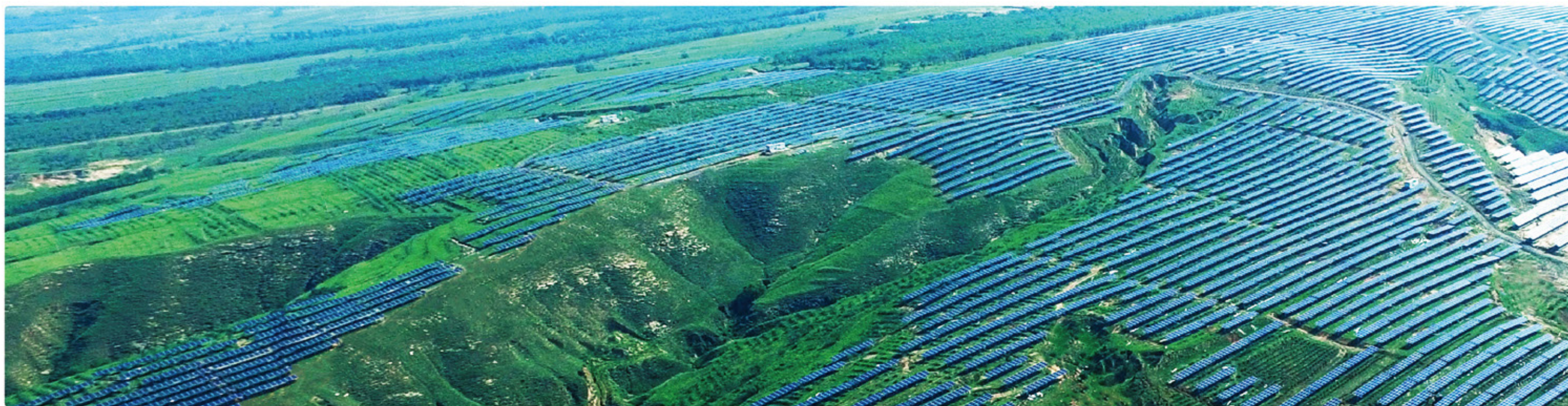
中国首个“光伏领跑者”计划项目——“山西大同采煤沉陷区国家先进技术光伏示范基地”50MW光伏电站 China's First "PV Leader Program" Project - "Shanxi Datong Coal Mining Subsidence Area National Advanced Technology PV Demonstration Base" 50MW PV Power Plant
