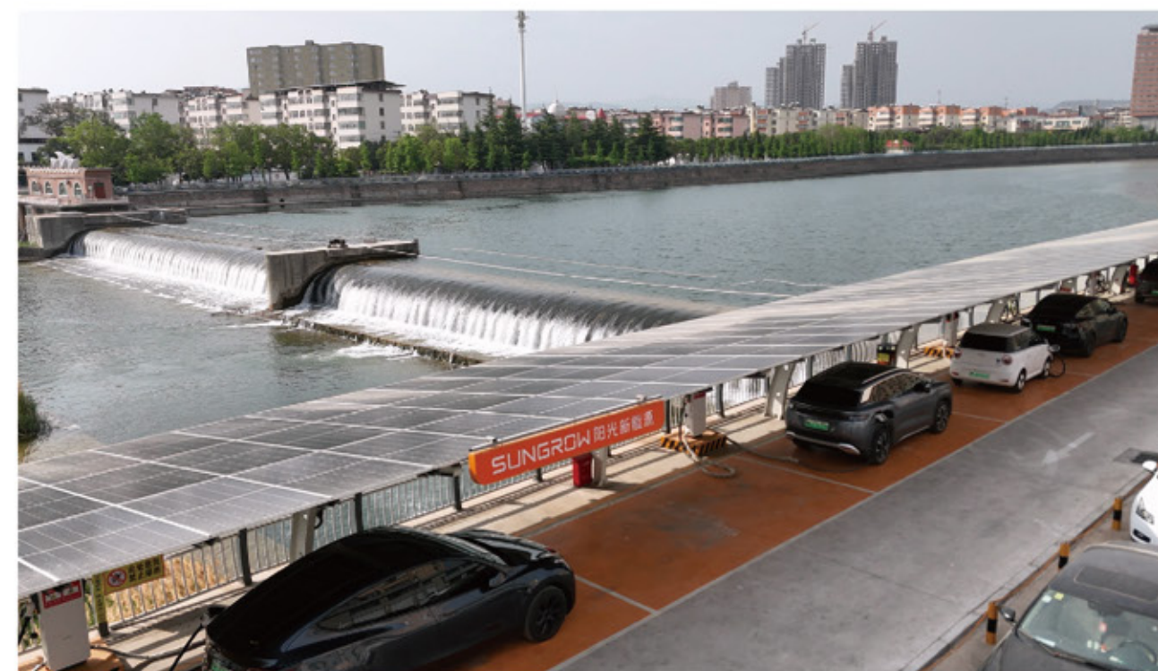
河南三门峡光充电站 Henan Sanmenxia PV-Charging Station
